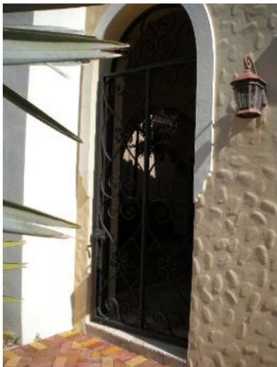
Grounds Gate Condition
