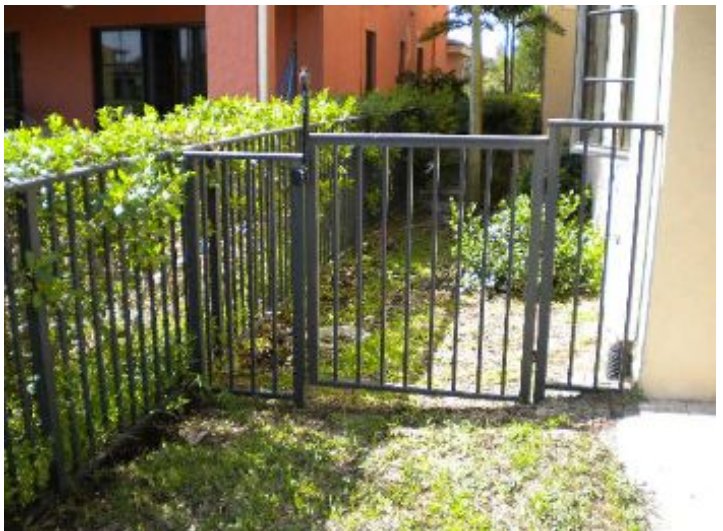
Grounds Gate Condition
