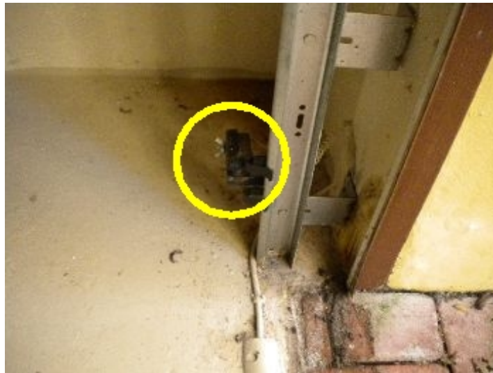
Eye beam system present and operating.
