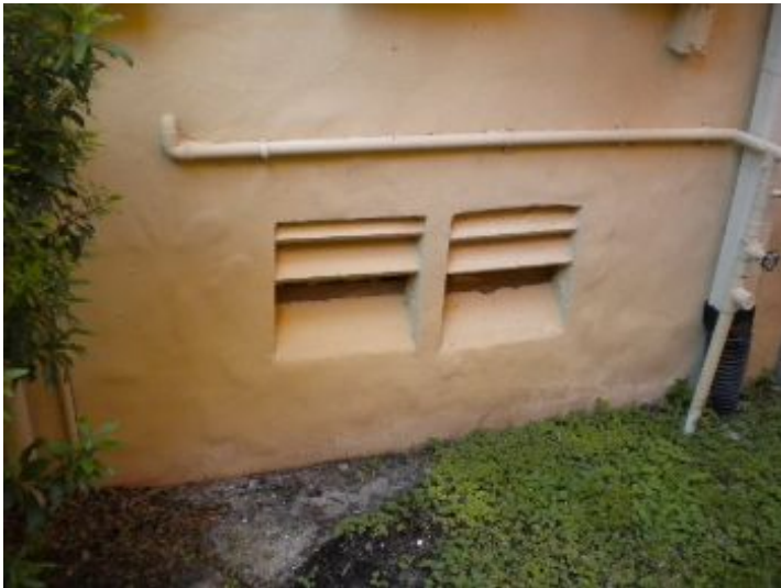
Vent located at bottom of East & West wall.
