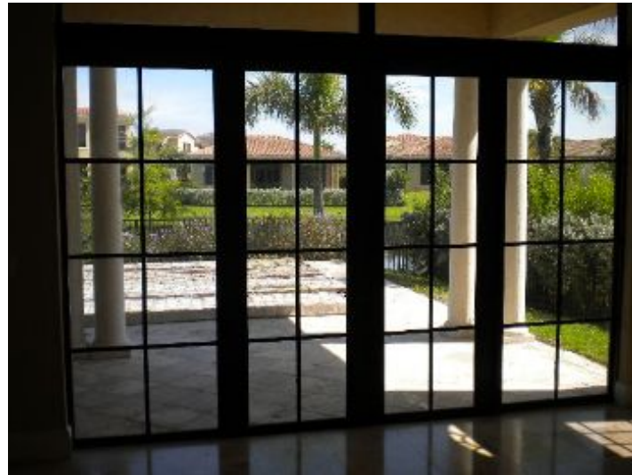
Interior Areas Patio Doors
