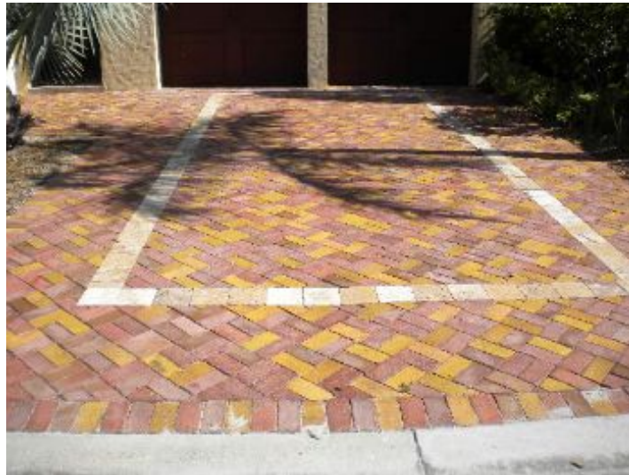
Grounds Driveway and Walkway Condition
