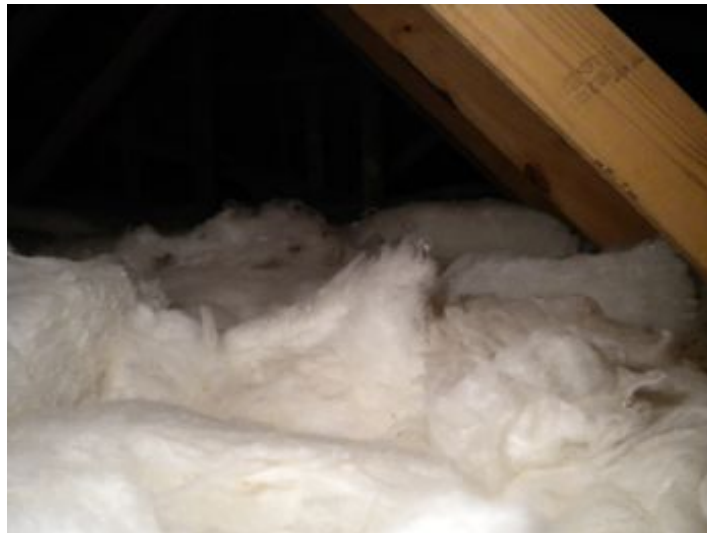
Attic Insulation Condition
